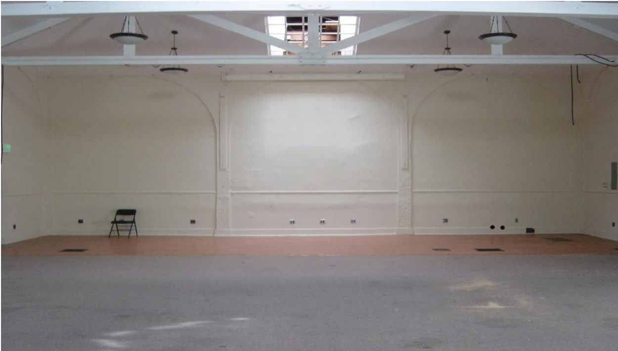
PHOTOGRAPH 2: VIEW OF THE INTERIOR OF THE FIRST FLOOR OF THE VACANT CHURCH.
