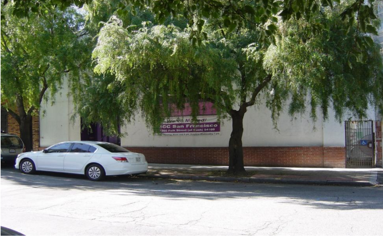
PHOTOGRAPH 1: VIEW OF THE VACANT TWO-STORY CHURCH FROM EUREKA STREET, LOOKING WEST.
