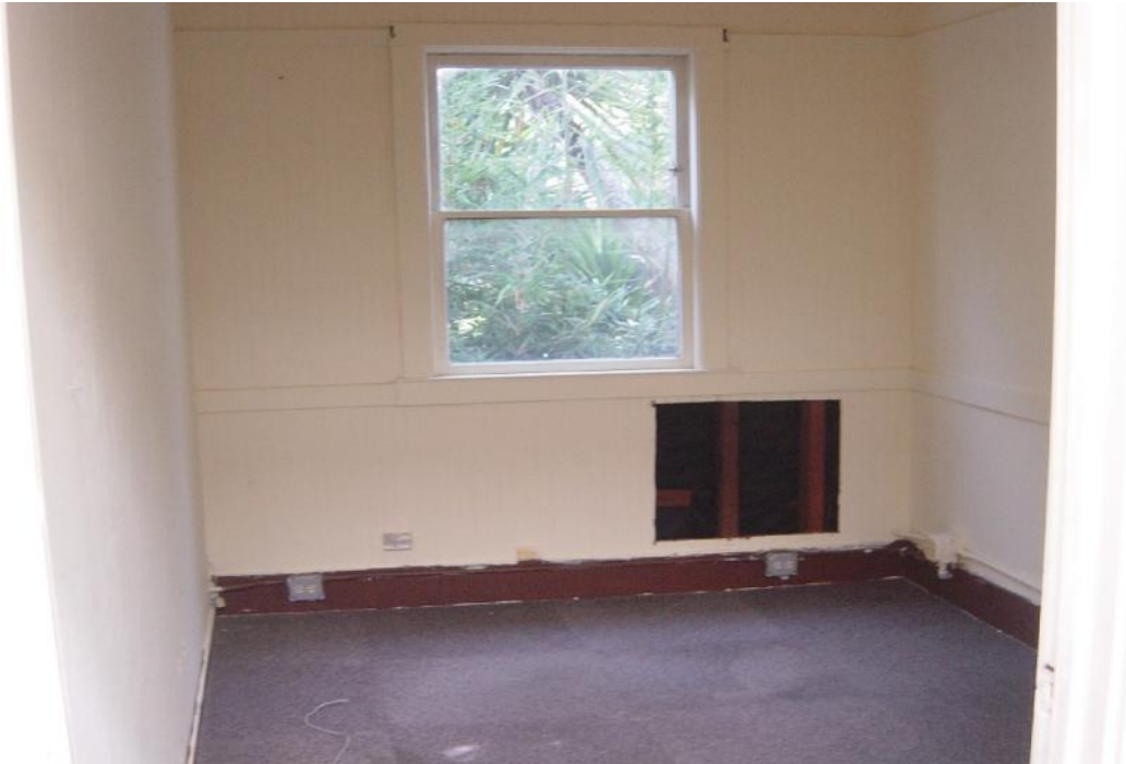
PHOTOGRAPH 5: VIEW OF THE INTERIOR OF THE SECOND FLOOR OF THE VACANT CHURCH.
